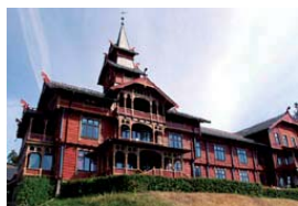
Holmenkollen Park Hotel, Oslo
