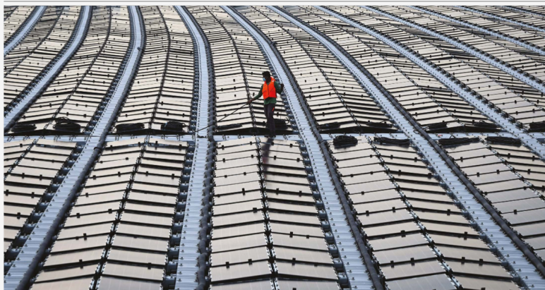
A worker tends to a floating solar-panel farm off the northern coast of Singapore.
