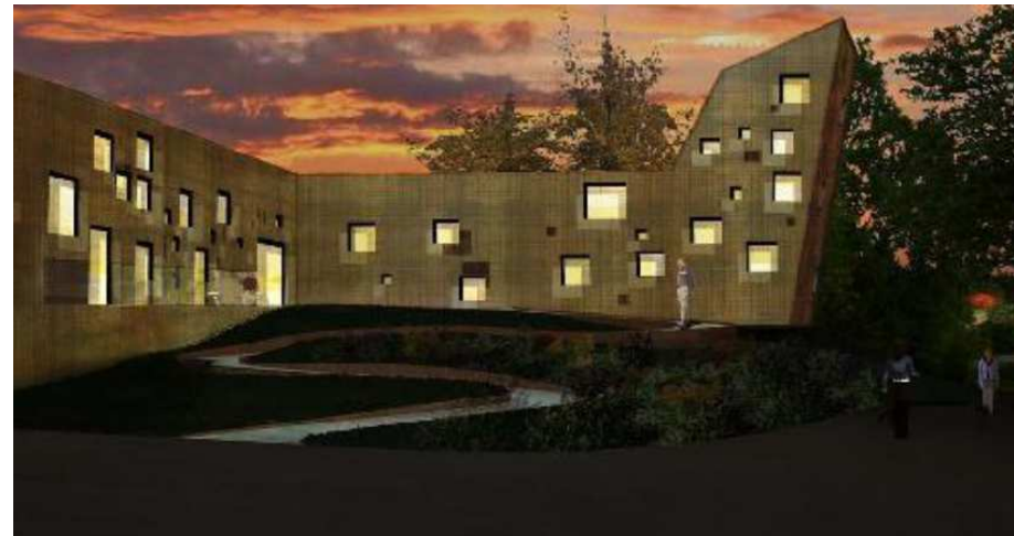
The new building for The Meteorological Institute by Arkitekt PIR II (work in progress)–the first By- og boligutstilling project in Oslo
