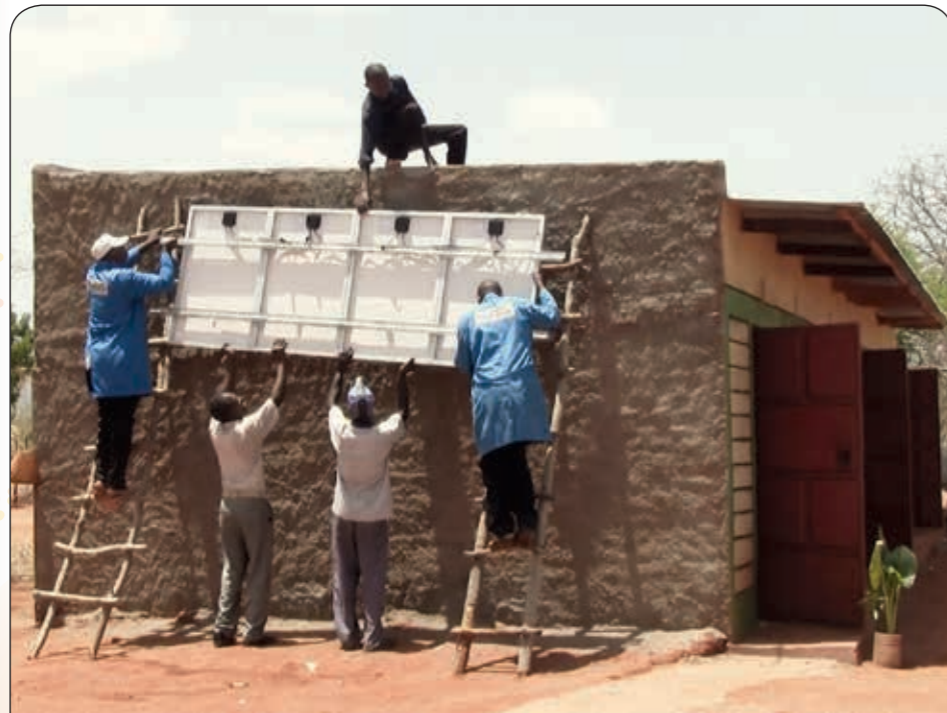
Carefull lifting of the Solar PV panels Photo: Marius Grøtvedt
