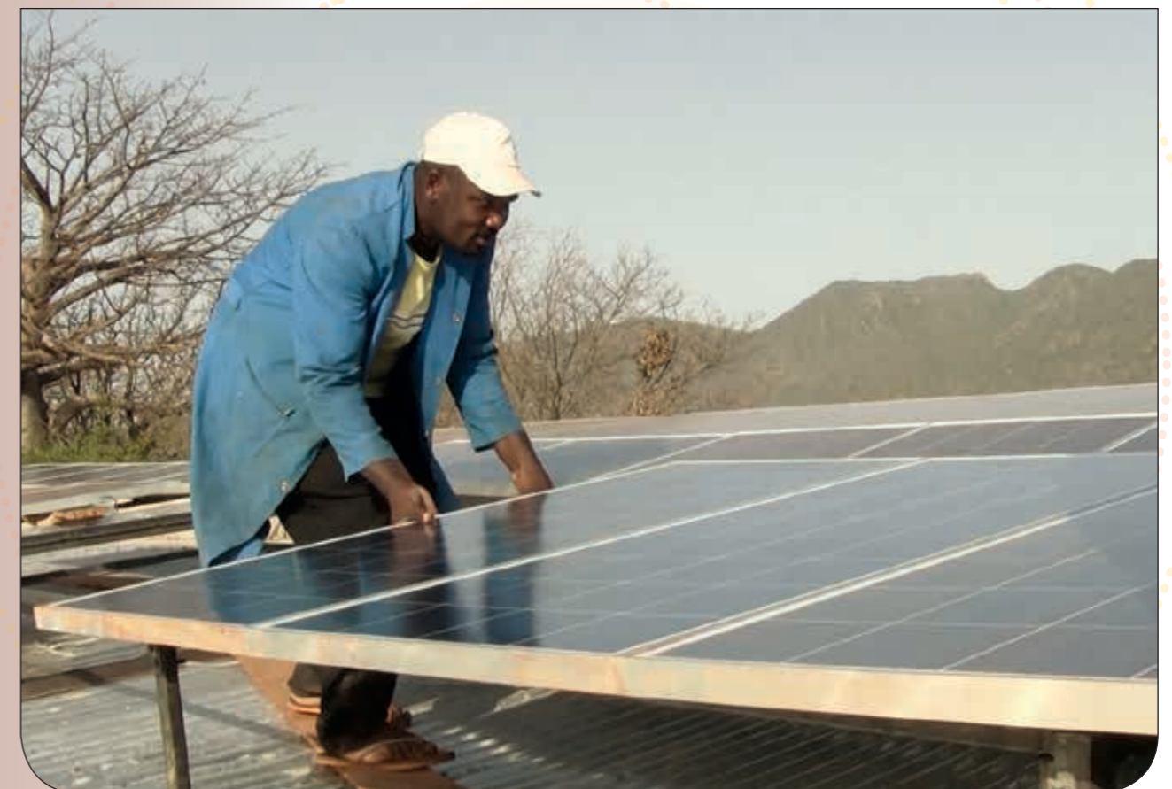
Installation by experienced technician Photo: Marius Grøtvedt
